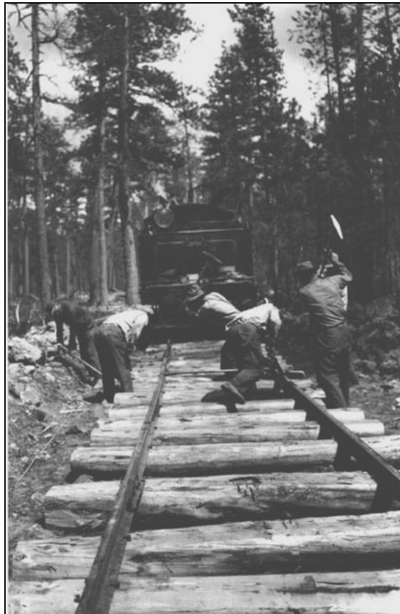
Figure 2 US forest service photo of crews laying track south of Bend.
